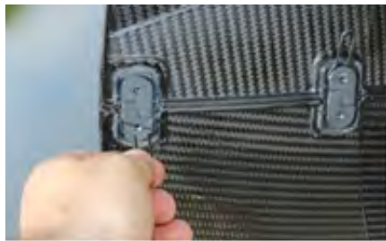
Figure 3-5: Latches to interconnect the panels
